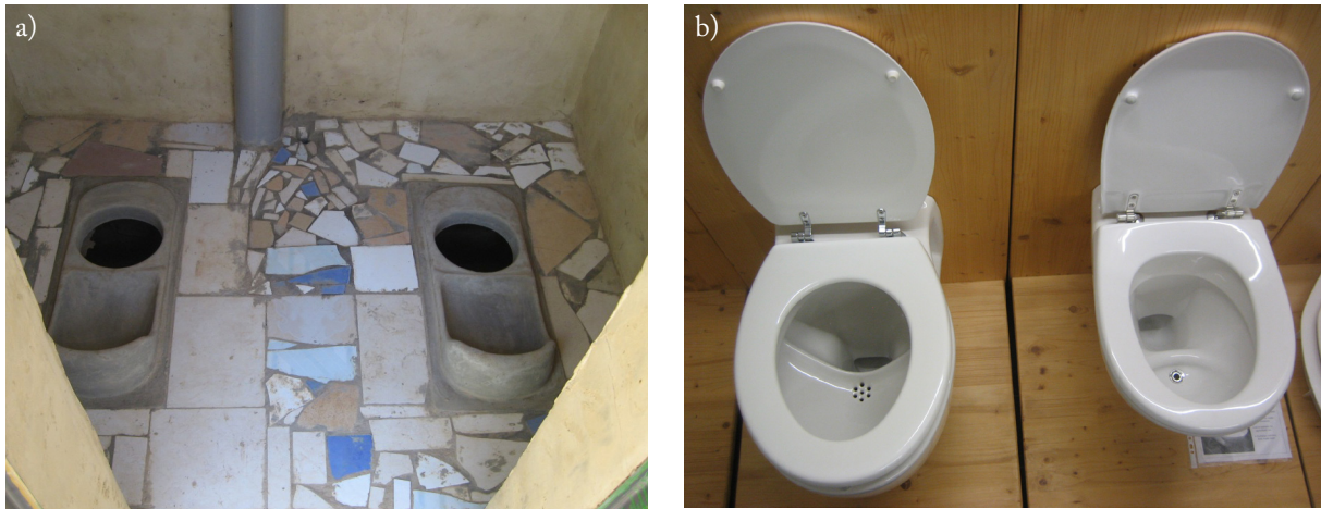
Figure 6.4 Urine, free from faecal contamination, can be used as a safe source of phosphorus fertiliser for crops. a) Urine diverting toilets in Nepal. Urine is collected in the basin at the front, whilst faeces collect in the hole at the back. b) Left: urine-diversion flush toilet by Roediger (Germany). A valve opens only when the user is seated to prevent flushing water from draining into the urine tank. Right: urine diversion flush toilet by Gustavsberg (Sweden). In this design no valve is used, this allows a little bit of flushing water to enter the urine pipe to avoid potential clogging of assemblies. Photographs courtesy of The Sustainable Sanitation Alliance (SuSanA).
